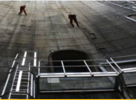
HYDRO-ELECTRIC DAM MAINTENANCE
