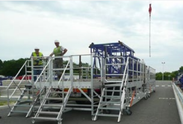
HOISTING, EQUIPMENT, STRUCTURAL WORK, BUILDINGS
