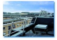
In the case of fixed guardrails, Tubesca-Comabi has designed three types of post supports: Z-shaped, platinum and surface-mounted to attach to various reception structures (parapets made of steel, concrete, stone or stringer). Once the type of fastening has been determined, it is also possible to select the type of post (straight or inclined) to preserve the building's aesthetic appearance.
