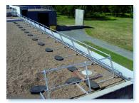
It is worth recalling that the use of free-standing guardrails is only possible on rooftops with a slope not exceeding 10°.
