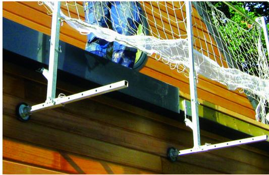
In addition to its Horizon range, Tubesca-Comabi also offers MOMENT'TOP products: temporary guardrails designed for work on rooftops and terraces, both new and renovated.
